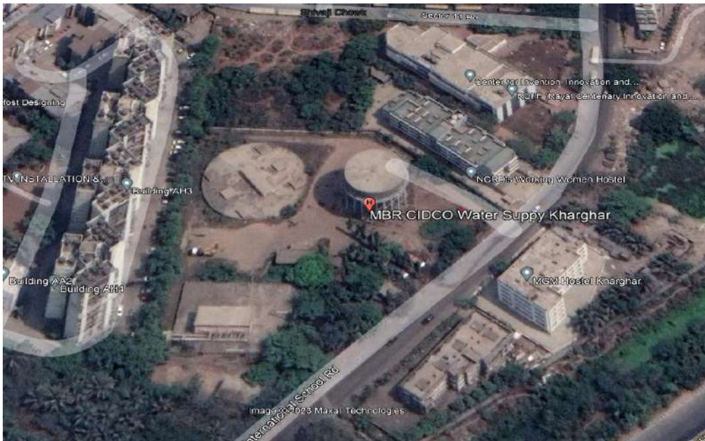
Figure 6.8: CIDCO Water Supply, Kharghar (19° 2'12.32"N, 73° 4'13.51"E)
