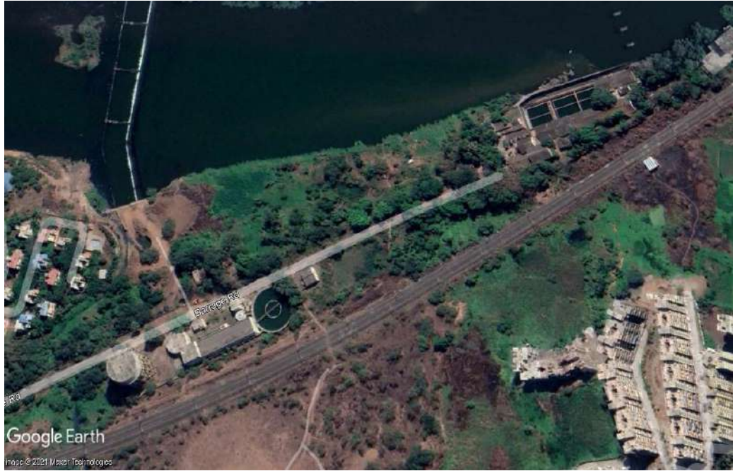
Figure 6.7: Badlapur Barrage Dam WTP (19°08'53.81" N, 73°15'09.89" E)
