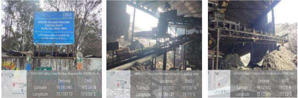
Figure 9.3: Wet Waste Processing Plant
