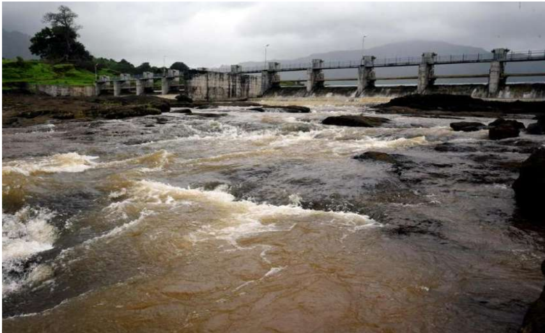
Figure 6.4: Dehrang Dam, Panvel
